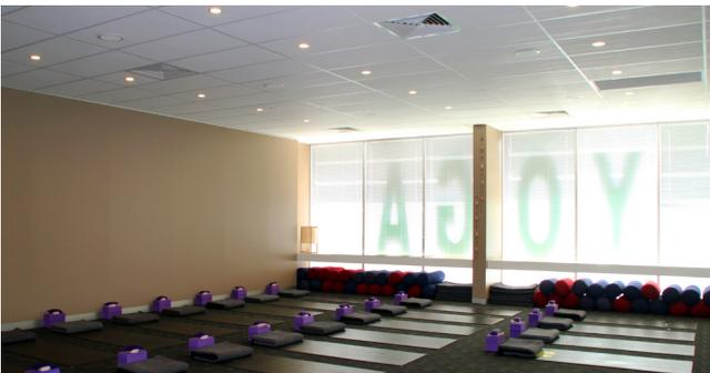
The glass walls and thin ceiling allowed intrusive noise to impact the comfort of the occupants
