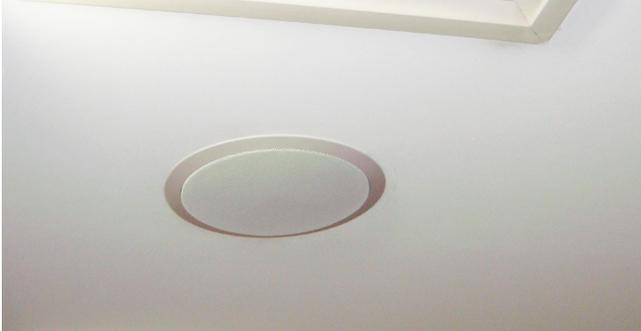
Soundmask's "cut in" transducer SM-TC-1265
