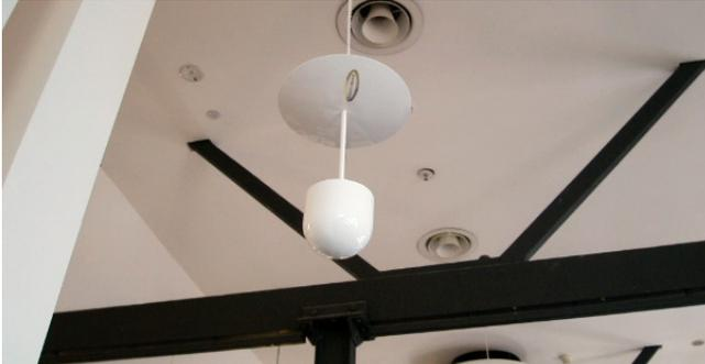
Soundmask transducer and acoustic disc in place
