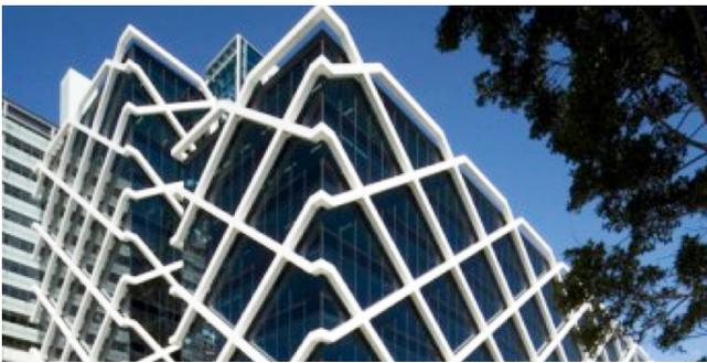
The building was designed with an asymmetric external diagrid
