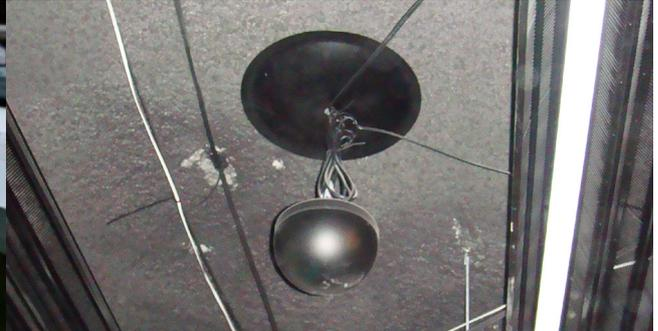
Installed transducer with acoustic disc
